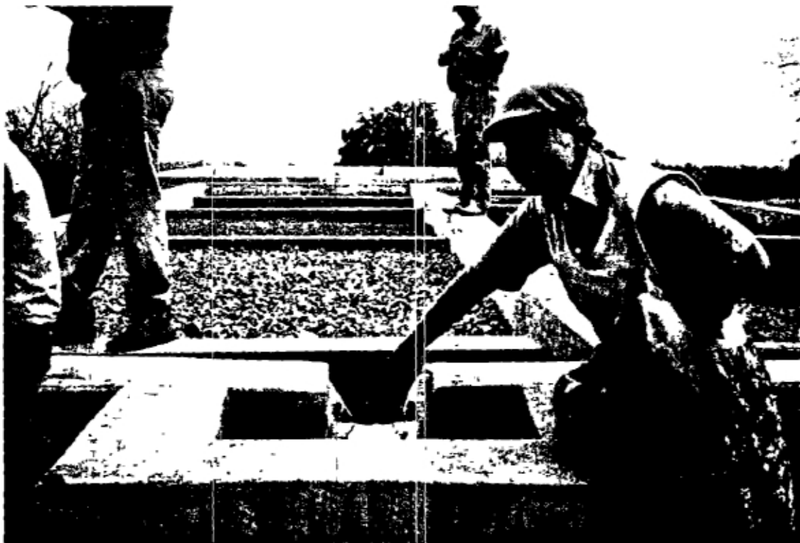
Wier at entrance to horizontal filters indicates low flows.
