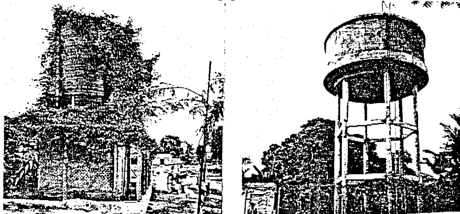
Reserves tanks and elevated tank
