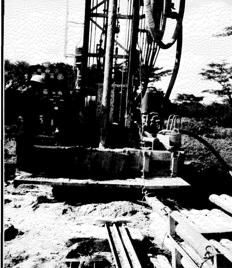
Drilling and borehole construction in Kiboga District
