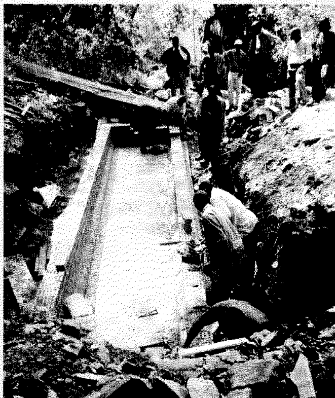
SSTWSP: Construction of sedimentation tank for Ibanda Water Supply System
