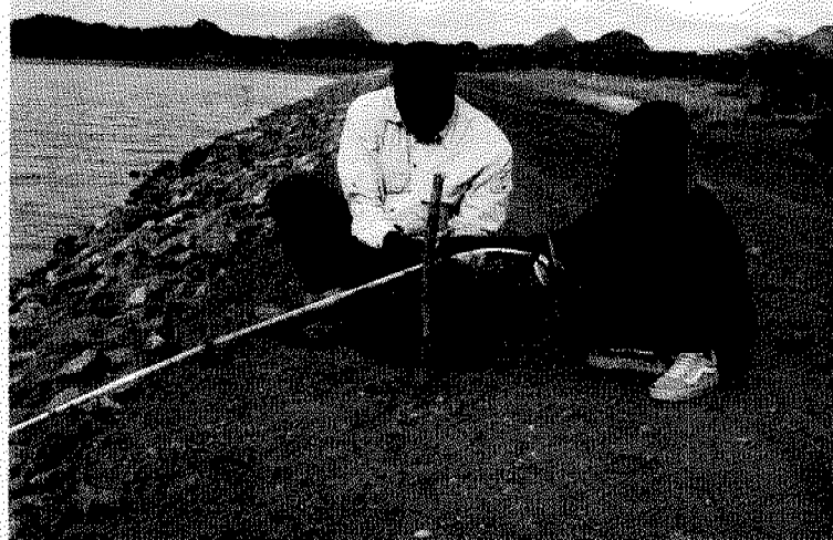
A senior engineer, Water for Production Unit, attesting embankment slopes during construction inspection of Longoritopoj dam, Jie County, Kotido District in 2002.
