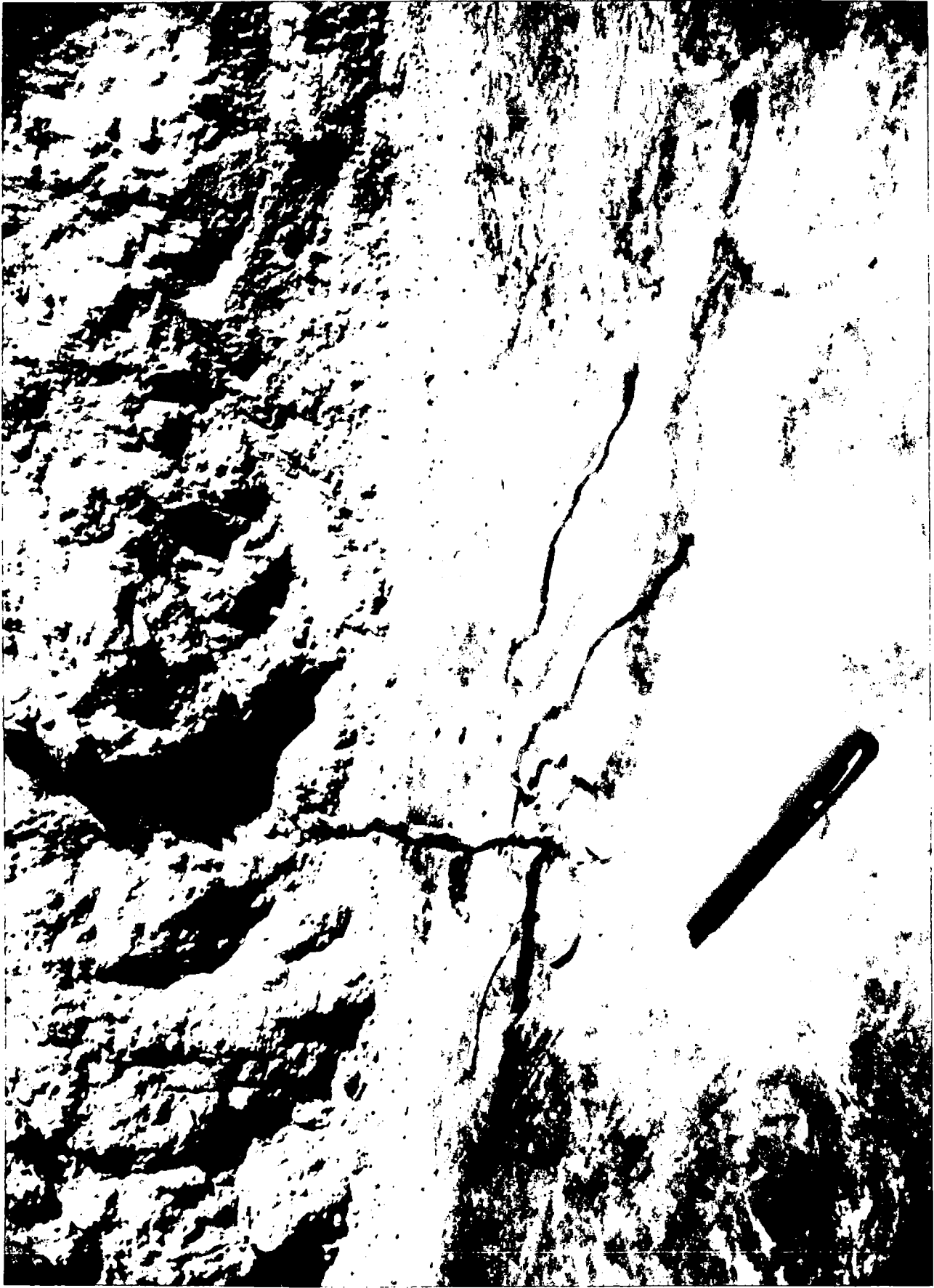
PLATE 11 Root growth through lining of hafir B
