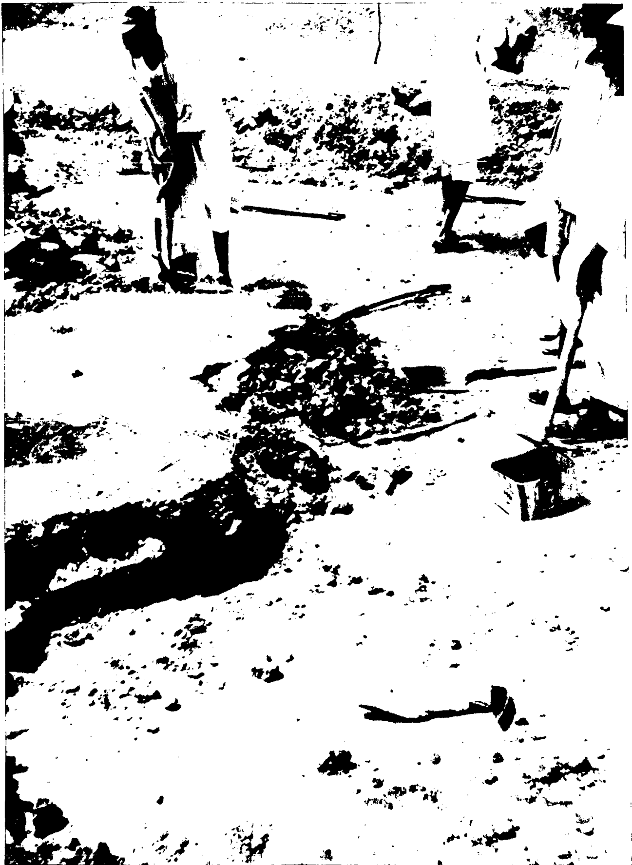
PLATE 3 Removing backfill from hafir A to expose polythene membrane
