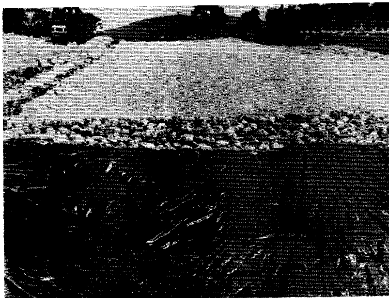
7. Trial Catchment programme; polyethylene with limestone aggregate.
