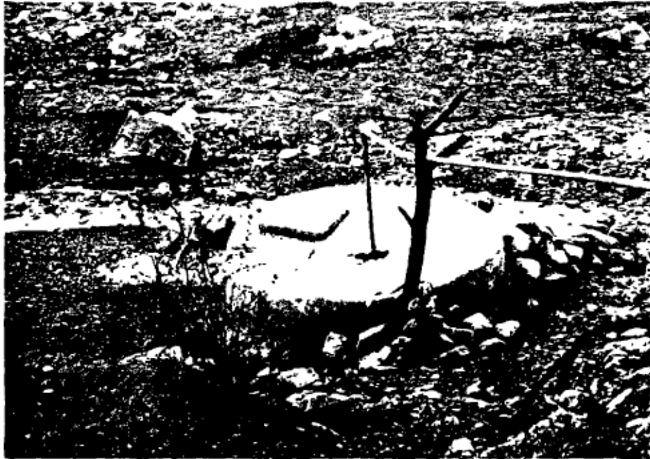
Photo 4. Well and unstable suction pipe, Carvajal, Chuquisaca.
