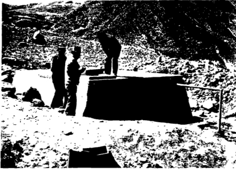
Photo 3. Typical water distribution system storage tank.
