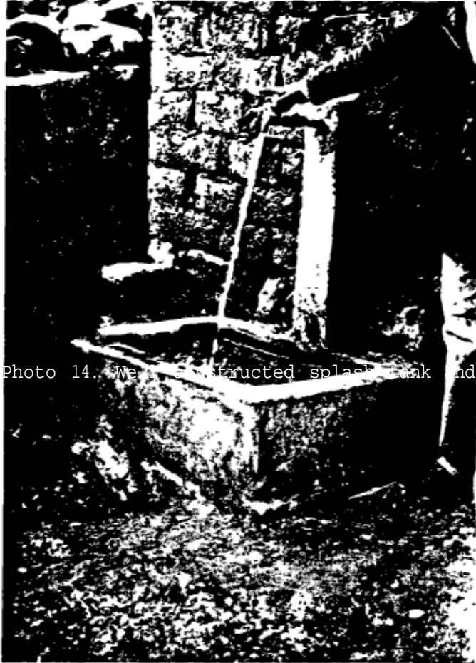
Photo 14. Well constructed splash tank and drainage.
