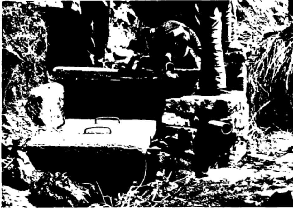
Photo 7. Intake structure subject to flooding and mud-slides, Copacabana, Oruro
