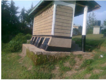
Dry composting toilets can be put in series
