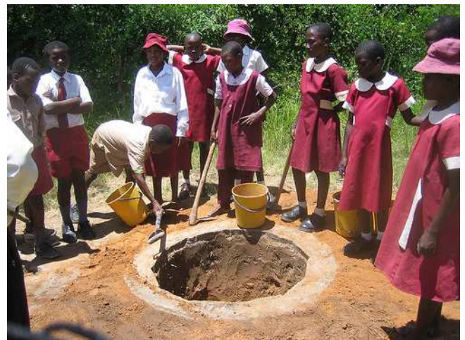
Figure 1: Pupils at a school in Epworth, Harare in Zimbabwe learn to build their own toilets: digging the shallow pit of an Arborloo inside a concrete ring beam (source: Aquamor). More photos of this school available here: http://www.flickr.com/photos/gzecosan/sets/72157626300000229/ .
