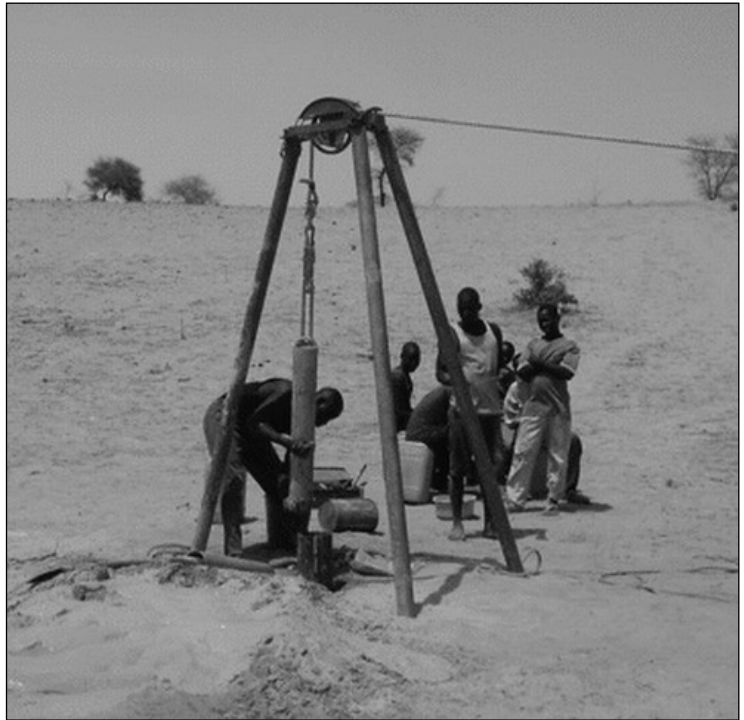
Figure 5. Hand percussion rig in action
