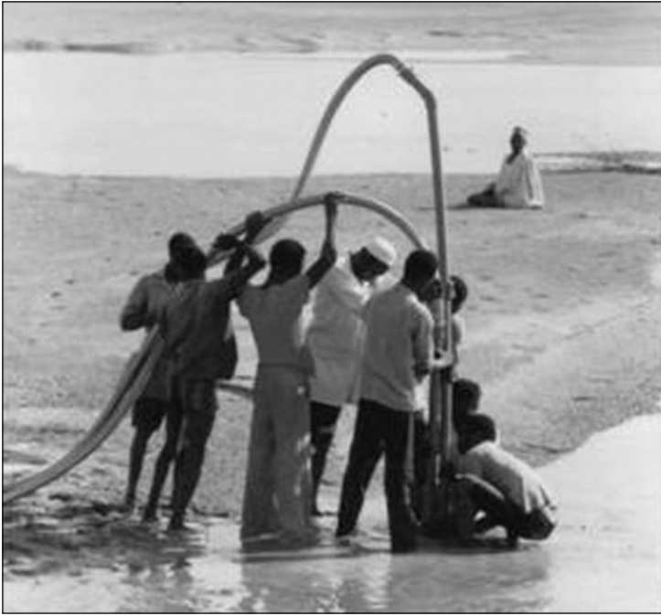
Figure 10. Well jetting in action
