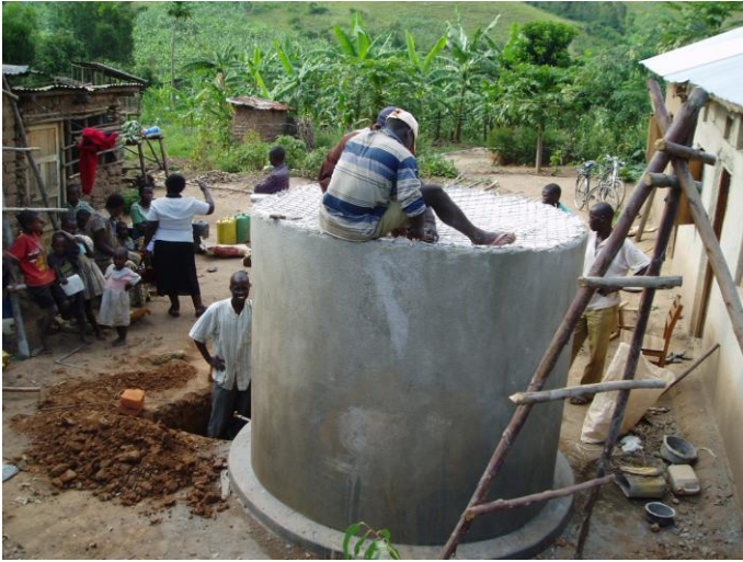
Figure 3: Construction of Ferro-cement Rainwater Tank
