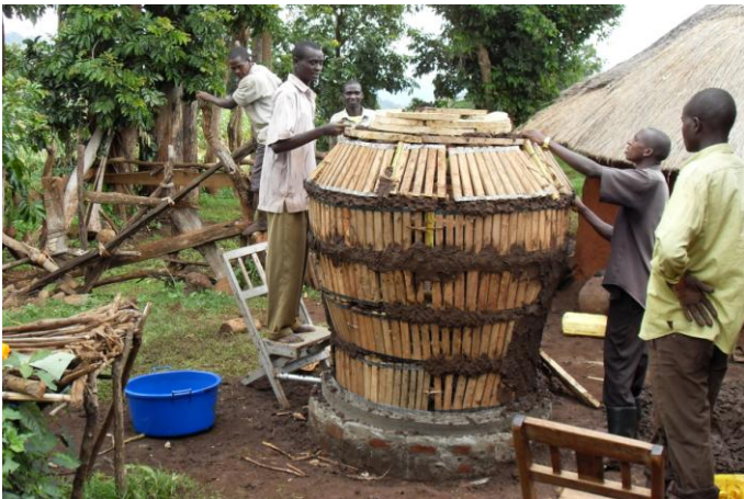
Figure 8: Rainwater Harvesting Jar under Construction
