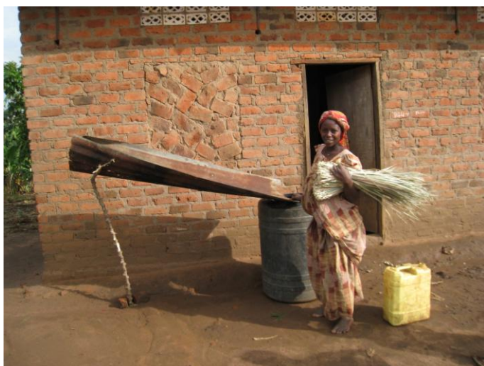
Figure 2: Typical informal Domestic Roofwater Harvesting
