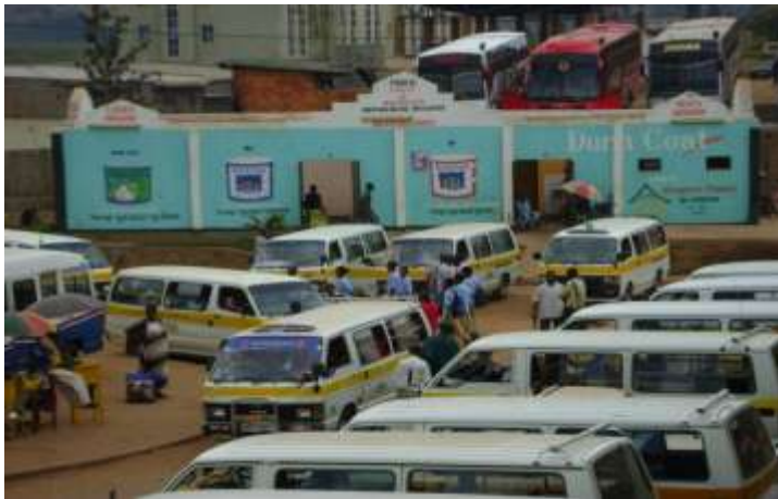
Nyabugogo car and bus parking eco-toilets
