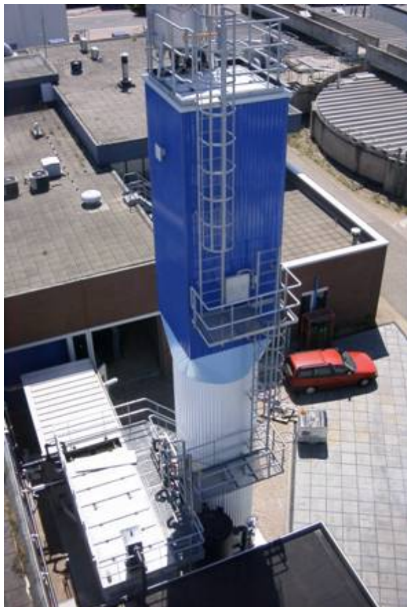
Figure 3. Schematic representation of the planned implementation of a combined sharon-anammox process for the removal of ammonium from sludge digestion effluent and picture of the demonstration anammox reactor of the icon EU research project at Rotterdam Dokhaven (Courtesy ZHEW and Paques).
