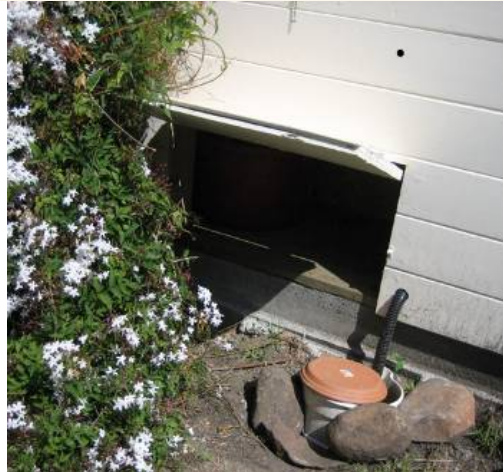
Figure 4: Urine and faeces collection from toilet in Figure 4.
