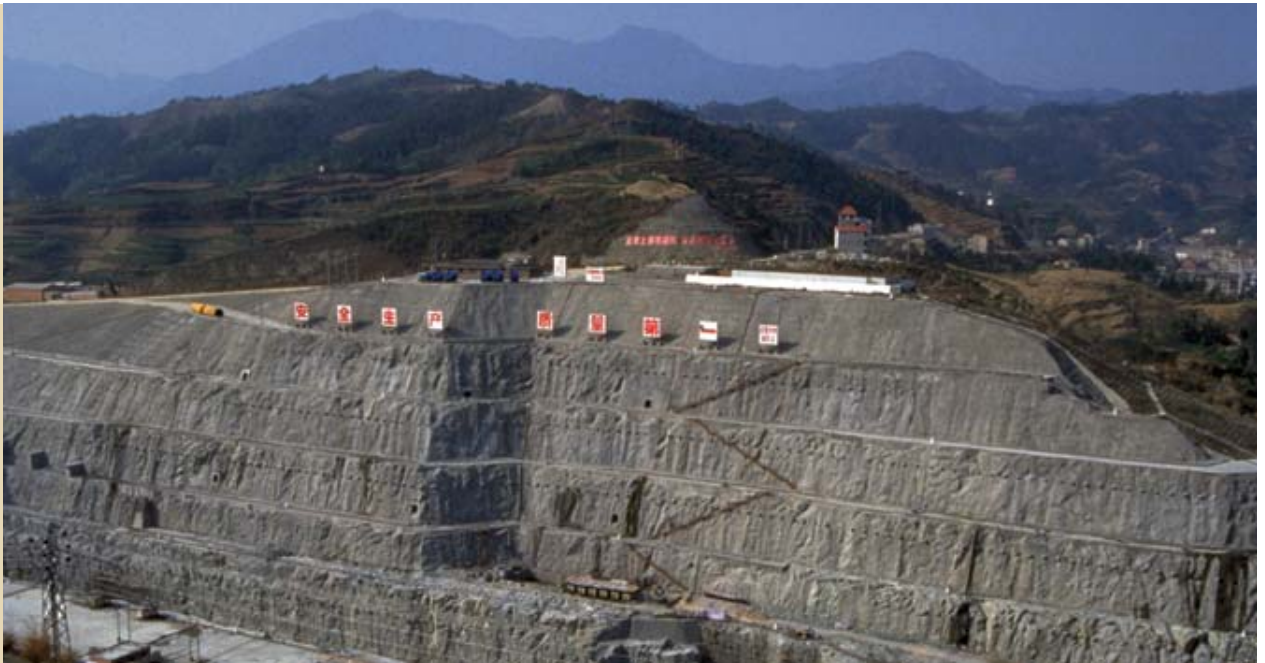
Three Gorges Dam, China.
