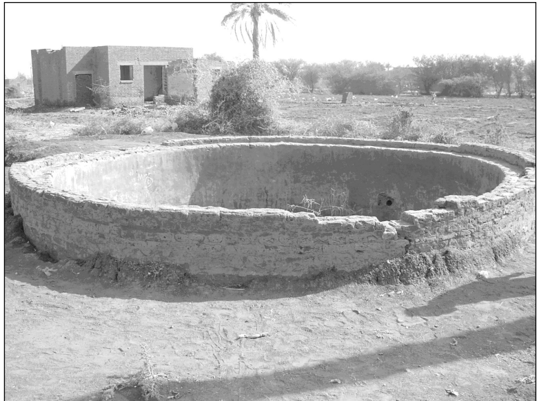
Non-functioning slow sand filter
