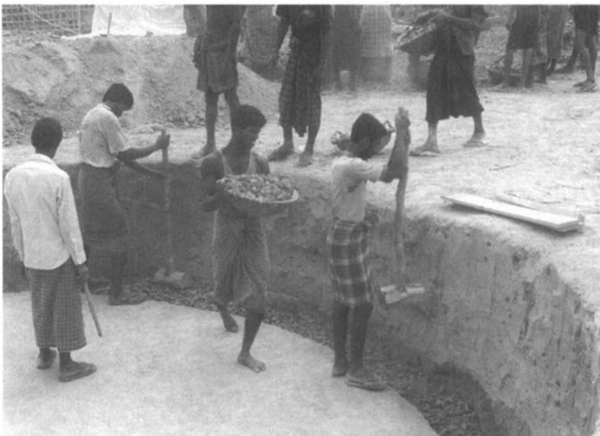
Preparing the tank foundations at Noyapara.
