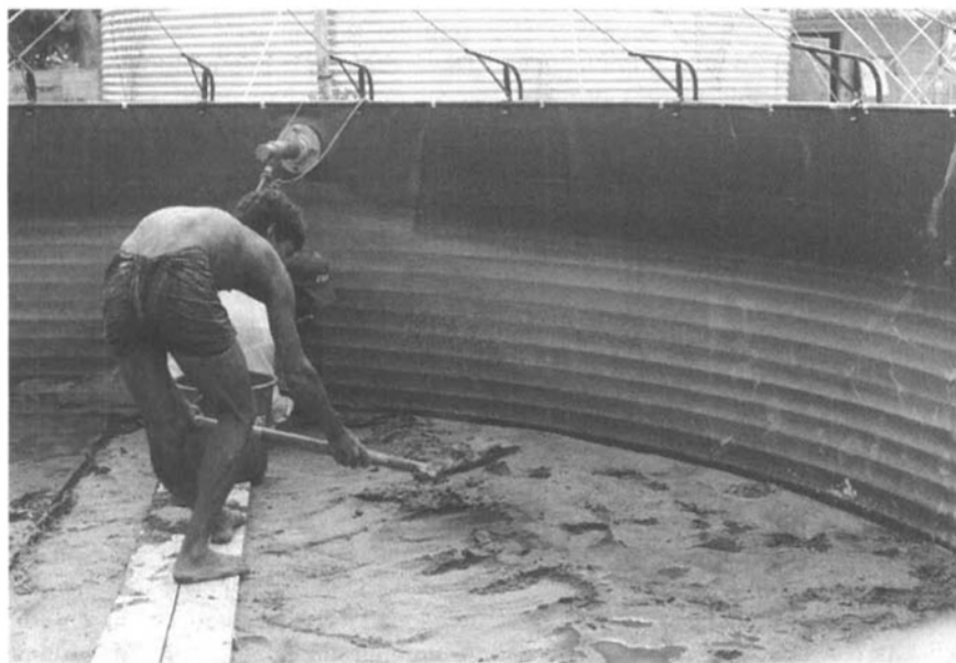
Skimming the 'slime layer' off a slow sand filter at Dumdumia.
