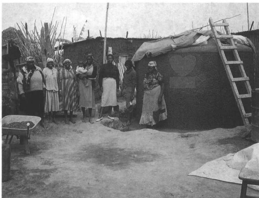
A women's group in Nakuru, Kenya, with their UNICEF-designed 12m 3 ferrocement tank.
