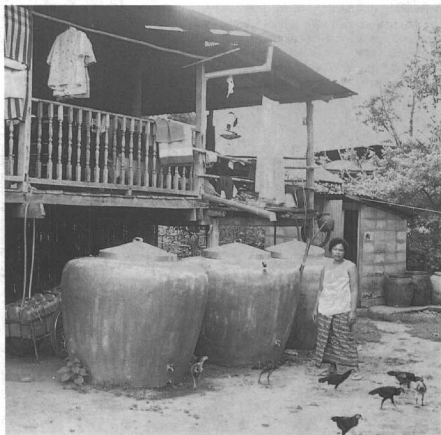
In Thailand alone more than 10 million 2m 3 ferrocement rainwater jars have been built since 1985.
