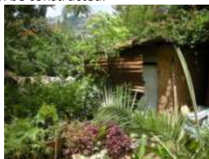
pic. 2 public pit latrine
