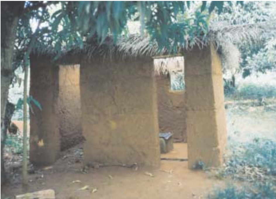
A new latrine under construction, using local materials, and adopted to incorporate a bath cabin.
