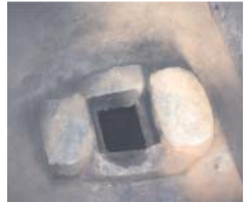
A customized pit latrine.
