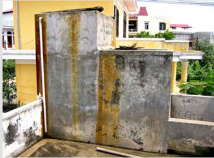
Figure 6. Sand filter installed on a house roof
