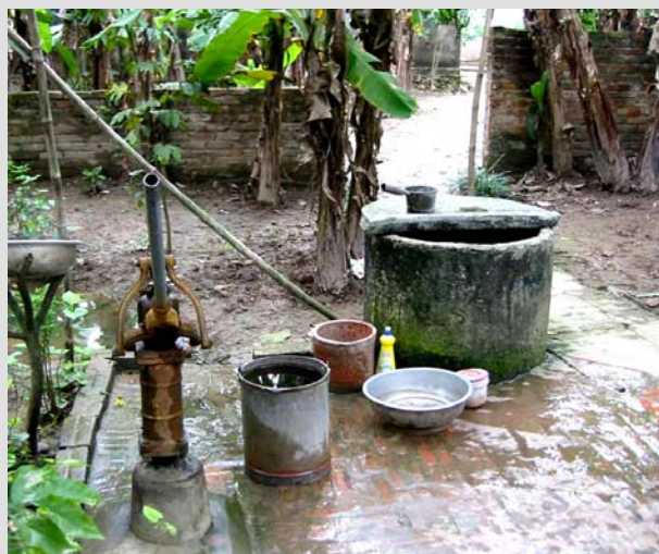
Hand pump and storage tank
