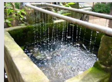
Figure 7. Aeration methods to enhance the oxygen supply in the sand filter:
