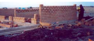
🏗️ Reinforced ground beam foundation supported by columns in Black Cotton soil.
