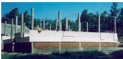
➡ The Poles and Rammed Earth construction process.
