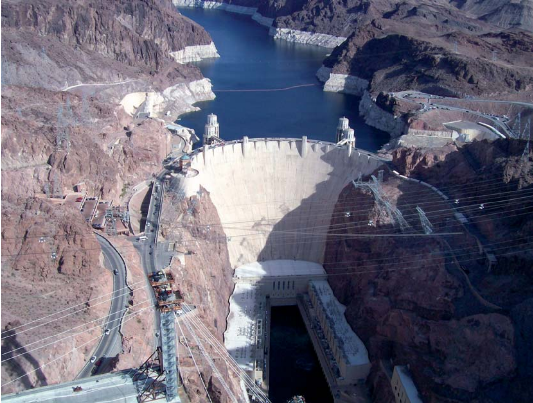
© Hoover Dam, USA.
