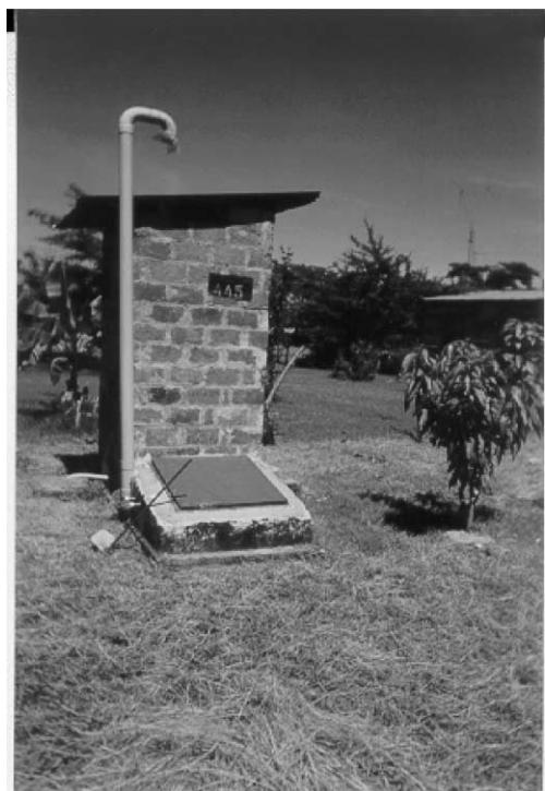
Figure 5 | Photographs of a double vault solar toilet in rural El Salvador.
