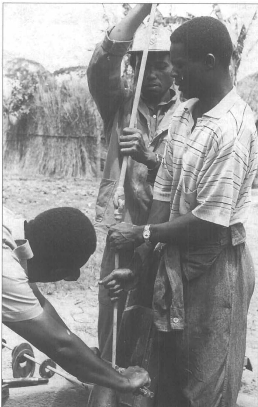
The 16mm rods are lifted one by one — stage 3 of replacing the seal.
