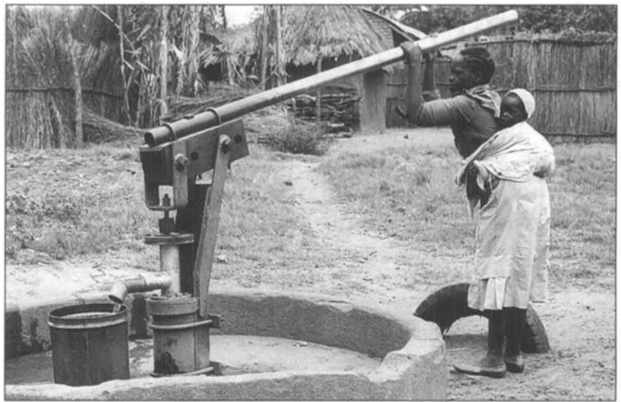
The Bush Pump undergoing trials at Idaho Farm in Norton, Zimbabwe.
