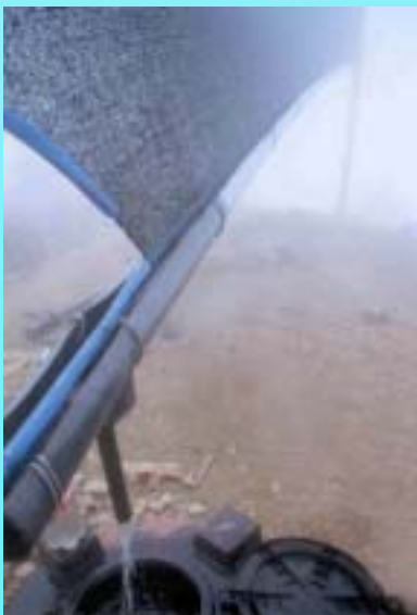
Fog water trickling down from the mesh and getting collected in the collection through, Dhojedanda, Dhankuta District
