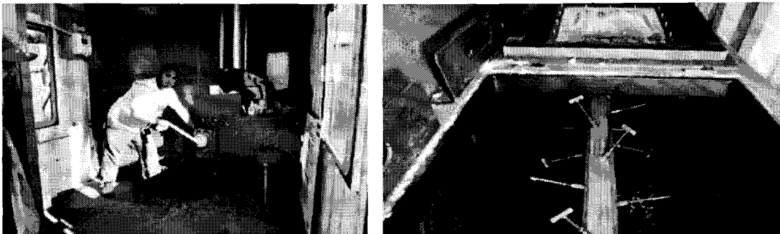
Figure 5 | Manual mixing device in caretaker room and second faeces chamber (separation panels can be seen in the left hand side).
