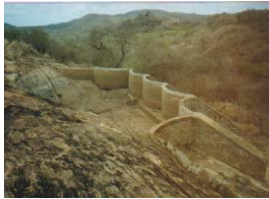
A multi-arch rock catchment dam built of concrete blocks on a rock shelf in Mutomo in 1985.
