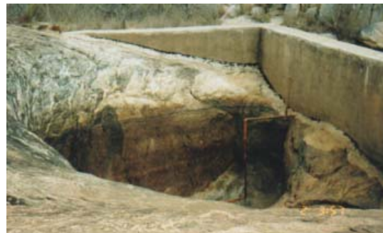
A V-shaped dam wall with a siphon pipe built around a rock pool at Mutomo
