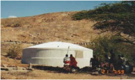
A rock catchment tank at Lakipia built by ASALCON Contractors in 1998.
