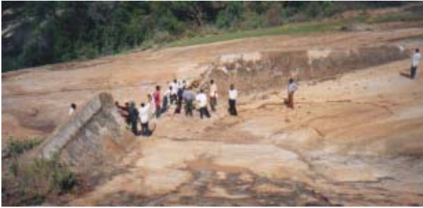
A dam wall filled with rubble stones packed in soil and covered with a coat of plaster was built at Kasiga in the 1950s. Twenty years later a large rock rolled down the catchment broke through the dam wall.
