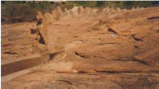
Garlands of stone gutters start their upward gradient (slope) of at least 3 cm per 100 cm from the end of a dam wall.
