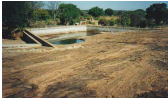
A dam wall with three sides built on a rock shelf at Kisasai, Kitui.
