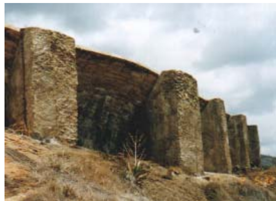
A multi-arch rock catchment dam built of concrete blocks on a rock shelf in Mutomo in 1985.
