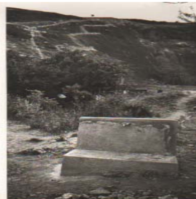
The pipe from the filter/intake box is mortared onto the rock until it reaches the tap stand.
