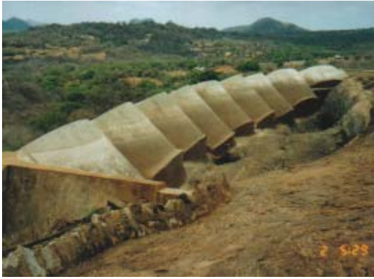
A slanting multi-arch rock catchment dam built of concrete blocks at Mutomo 1986.
