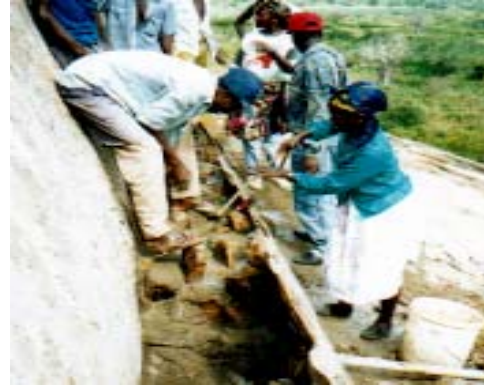
Detail of the second stage being built onto the first stage.
