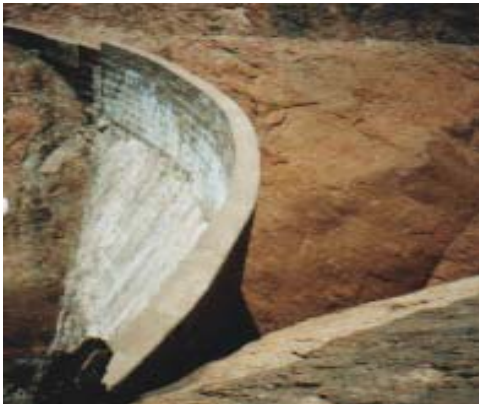
A single arch rock catchment dam built of concrete blocks in a gorge between two rocks in Mutomo in 1984.
