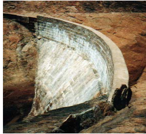
A single arch rock catchment dam.
