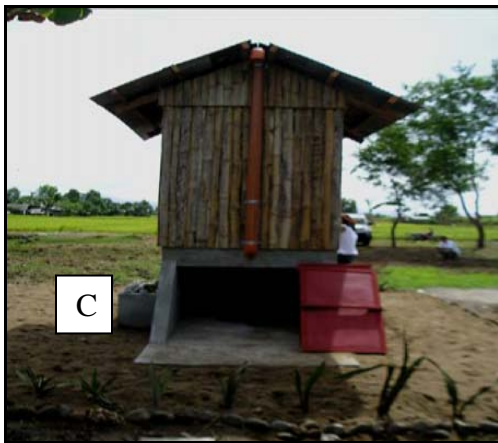
Figure 7.15: Designs that would make the emptying easier at small scale
