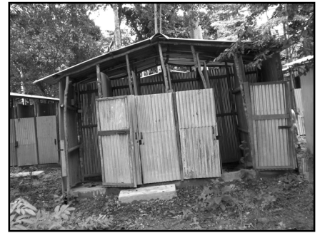
These toilets had been abandoned
