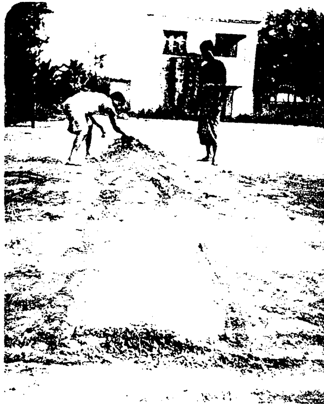
Bases is being prepared with sand for casting of segment of 3200 litre Tank.
