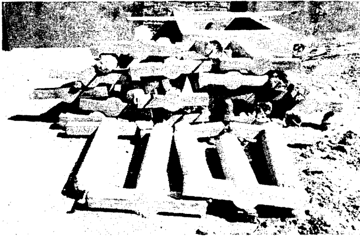
Ashrafpur scheme; stock of prefab public standposts
