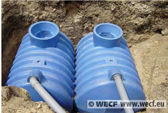
Figure 22 Example of underground with plastic urine storage tanks at Gradanitsy school in Ukraine (photo by WECF 2010)
