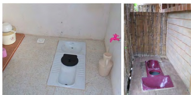
Figure 11: Left: Model from Shital Ceramics (India) installed in Afghanistan. Right: Reversible pan from Systems in N-Fibro in Rajajinagar, India
