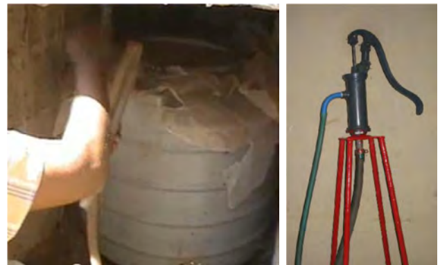
Figure 23 Manual withdrawal from above ground tank via hose pipe in Sodo, Ethiopia and piston pump from underground tank in India (photo by rosafrica (account youtube) and S.M.Navrekar, 2010)
