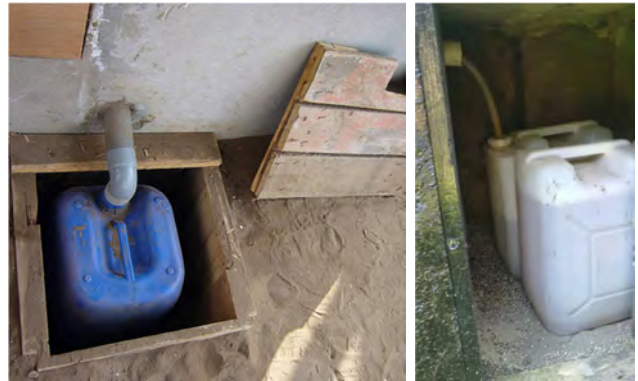
Figure 21 Examples of urine piping into jerrican Left: underground location with PVC piping in Peru. Right: above ground collection from hose pipe in extra chamber in Zambia (photos by H. Hoffmann, 2009 and R. Ingle 2010)
