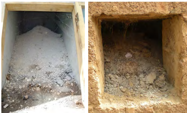
Figure 28 Examples of dried faeces covered with ash inside the vault in the Philippines and a soil and ash mix in Burkina Faso (photo by E. Sayre, 2008 and S. Tapsoba 2009)
