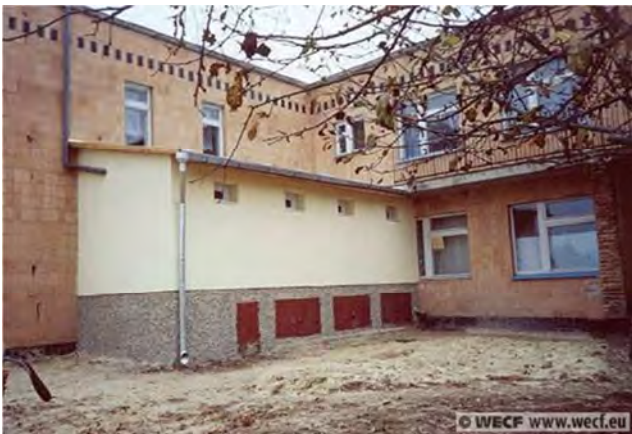
Figure 35 UDDTs in schools are attached to school building so that students can enter the restrooms from indoors, Ukraine (photo by WECF, 2006)
