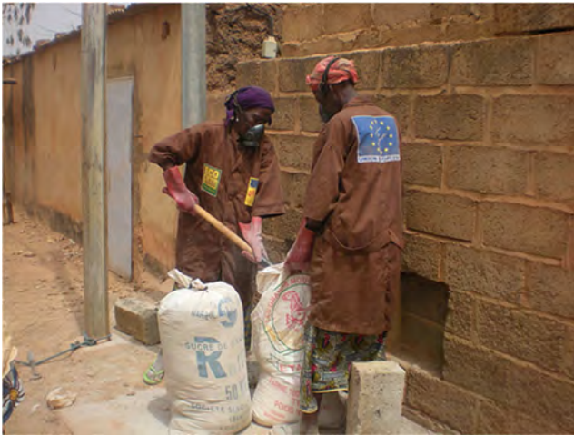
Figure 32. The inactive vault is manually emptied after a storage of 6 months and then taken to external treatment stations for another 2 months of dehydration prior to reuse, Burkina Faso (photo by S. Tapsoba, 2009).
