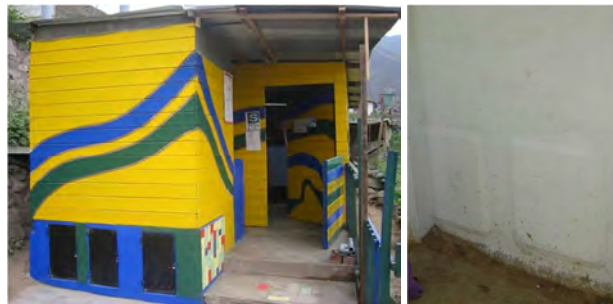
Figure 17 Example of metal vault doors with looks at a school in Lima, Peru and semi-permanent doors made from concrete slabs at a household in India (photos by C. Olt, 2009 and Lucas Dengel, 2009)
