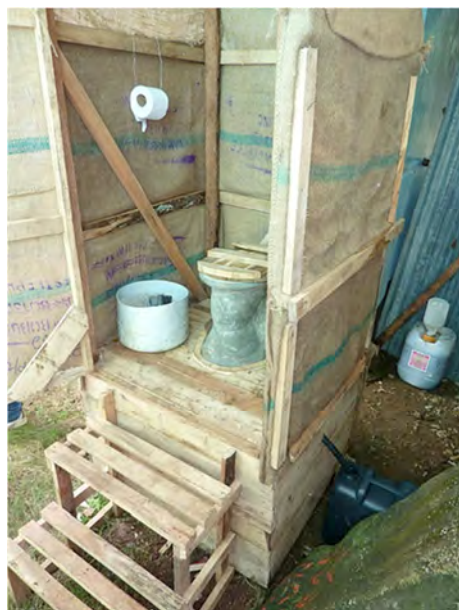
Figure 33. Low cost model of a single vault system in the Philippines by WAND (photo by R. Gensch, 2009)
