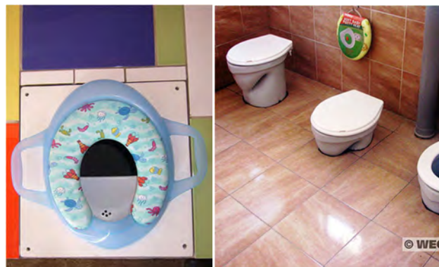
Figure 27. Use of a movable seat adapter in Peru and sunk in UD pedestals in Georgia (photo by H.Hoffmann, 2009)
