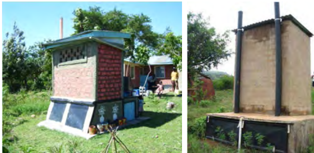
Figure 18: Left: UDDT with slightly inclined metal vault doors in Chwele, Western Province. Right: Toilet in eThekweni (Durban) in South Africa with vertical and sideways sliding plastic doors (photos by C.Rieck, 2010 and EWS, 2009)
