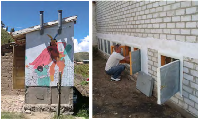
Figure 15. Double vault UDDT in near Cusco in Peru and at a school in Nizhyn in Ukraine (photo by H.Hoffman and WECF)
