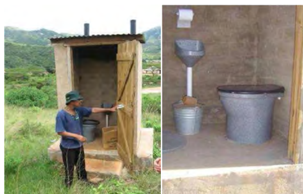
Figure 34. Peri-urban UDDTs constructed by eThekweni municipality on large-scale (photo by EWS). See also Figure 18.
