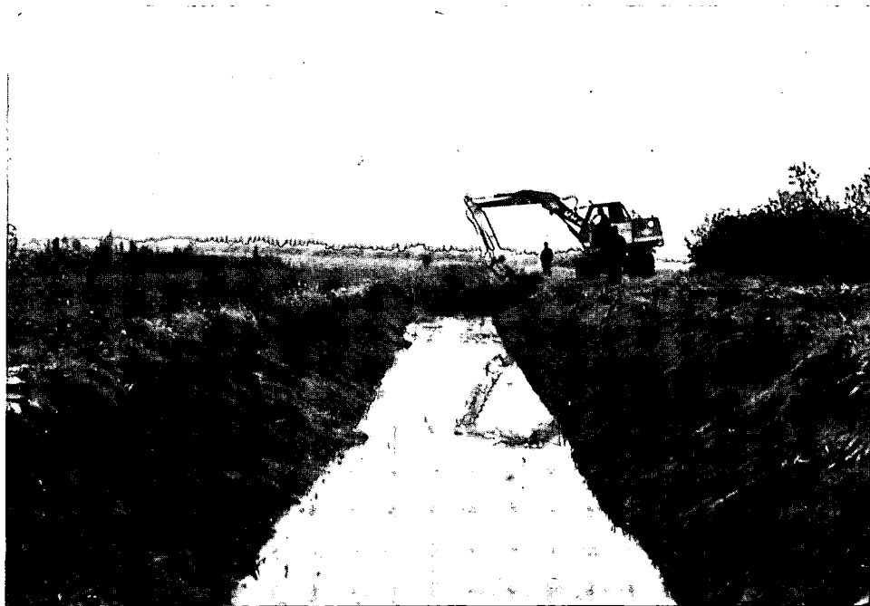
Photo 19.3 This machine can clean a drain with this top-width by working from one side only.
