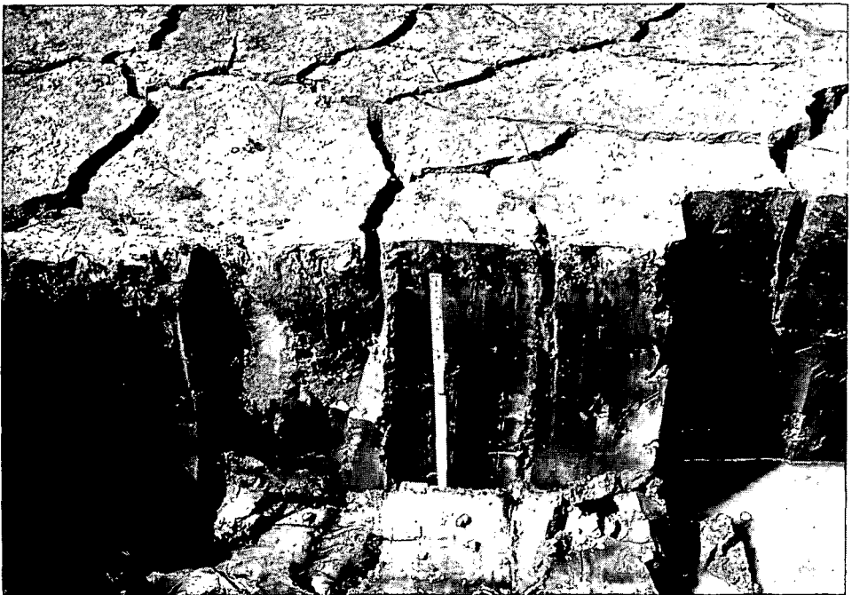
Figure 13.8 Crack formation in a recently reclaimed soft soil (De Glopper 1989)
