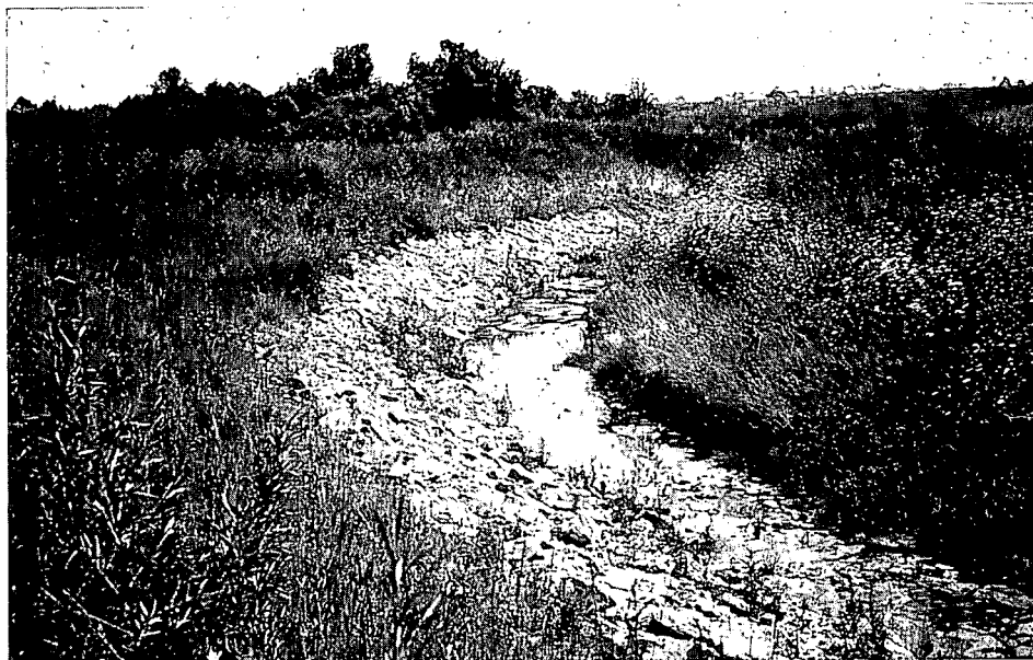
Photo 19.4 Local failure of side slope upon construction (courtesy, L Molenaar).
