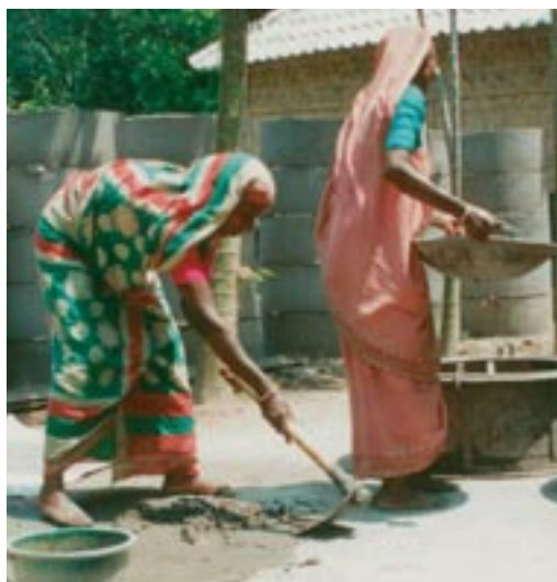
Concrete rings for latrine construction.
