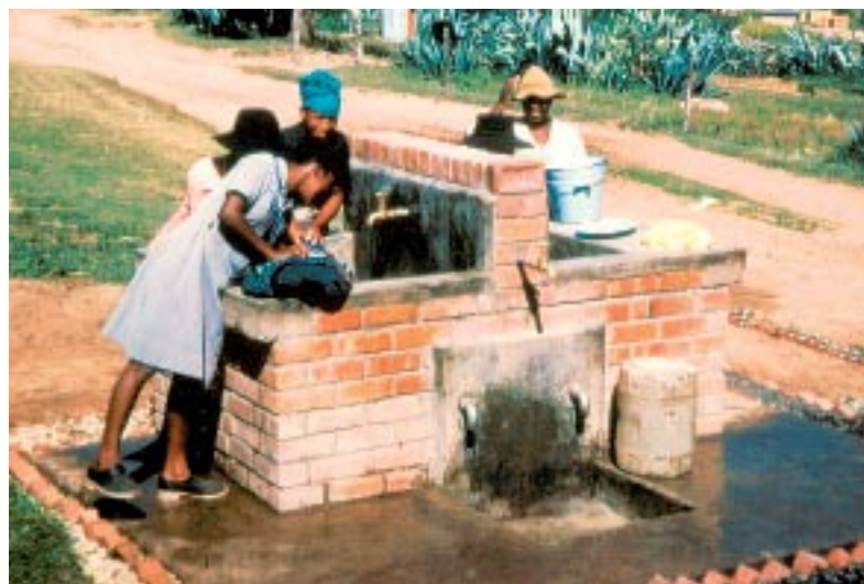
A facility combining standpipe and washstand.
