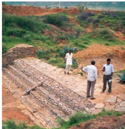
Measures for erosion protection and improved groundwater recharge using local materials.
