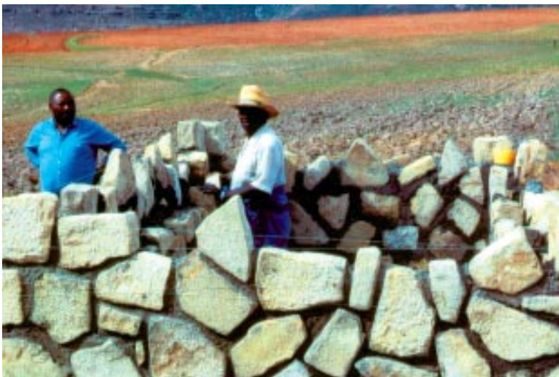
Building a water tank.
