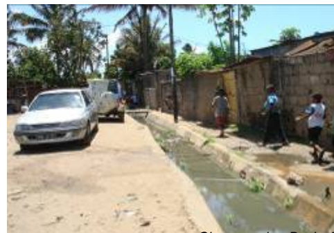
Chamanculo - Basin A Secondary storm water drainage channel
