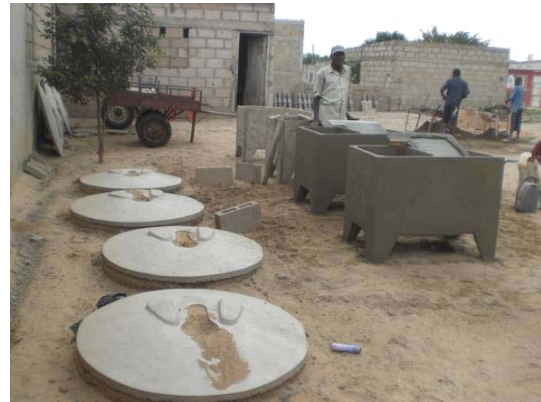
Locally made squatting plates use for improved latrines
