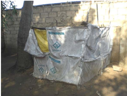
Commonly used latrine superstructures in underprivileged areas
