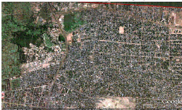
G – George Dimitrov: - Planned – Medium density residential areas with strong development along main roads. Limited water supply and on-site sanitation facilities
