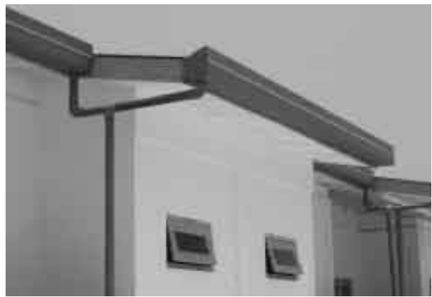
A house with a good gutter.
