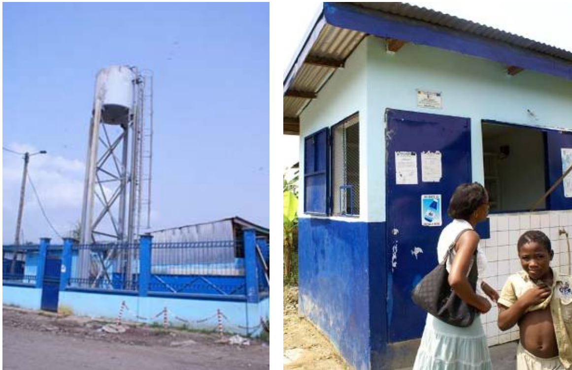
Figure 2.5 Communal water pump and local water treatment plant (Photo credit: Shaheed A, 2009)
