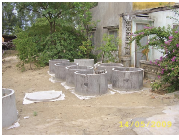
FIGURE 16: PRE-CAST RINGS FOR (SEMI) SEPTIC TANKS
