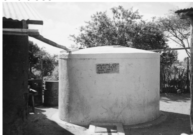
Fig. 1 Roof catchment and storage photograph by John Mbugua, Kenya
