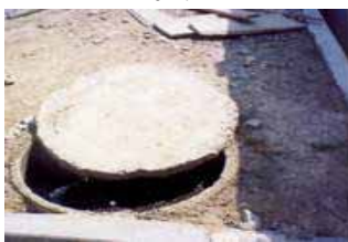
Covered disposal point of sludge
