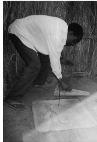
Figure 1b. Same latrine improved by installation of SanPlat Slab (Photo by EEPCO 2002)
