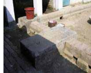
Sealed inlet facilitiv to add cow duna
