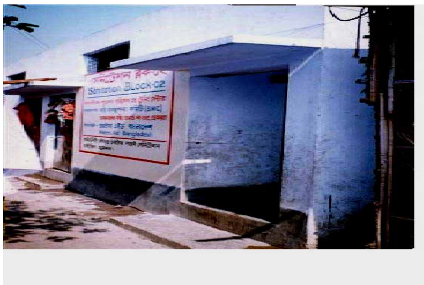
Figure 2. One Sanitation Block in Aynal's Bastee
