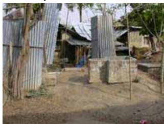
A community Biogas plant (human excreta based)
