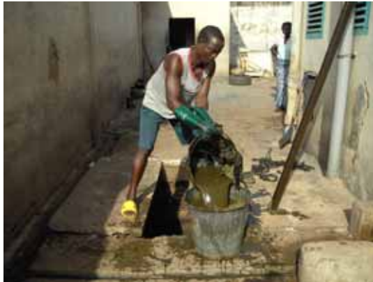
Figure 2. Manual emptying service provision by KMA/WMD in a house at Zongo, Kumasi (Photos: Anselme Vodounhessi)
