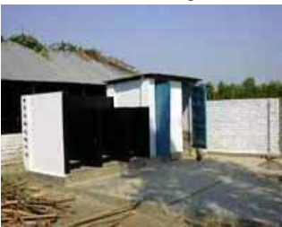
The biogas plant with inlets
