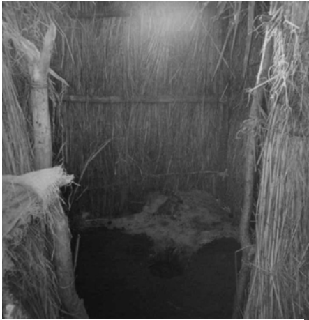
Figure 1a. Traditional pit latrine in Magugu Babati District Arusha (now Manyara) region. (Photo by EEPCO 2002)
