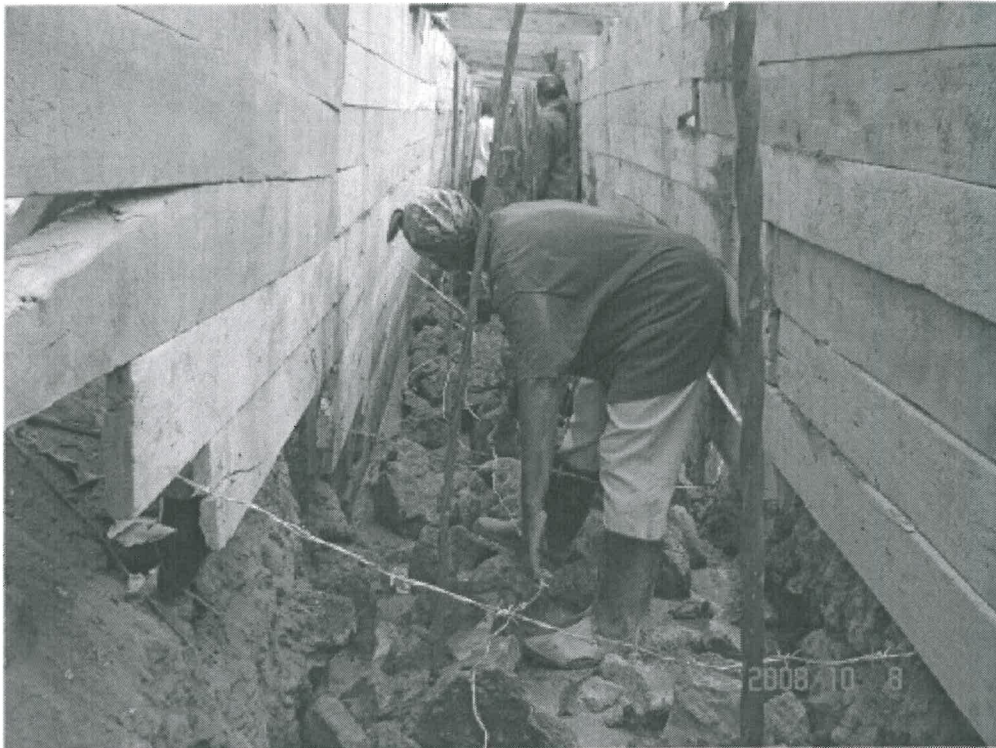
Figure 3: Artisan in trench showing form work, steel rebars, and barbed wire
