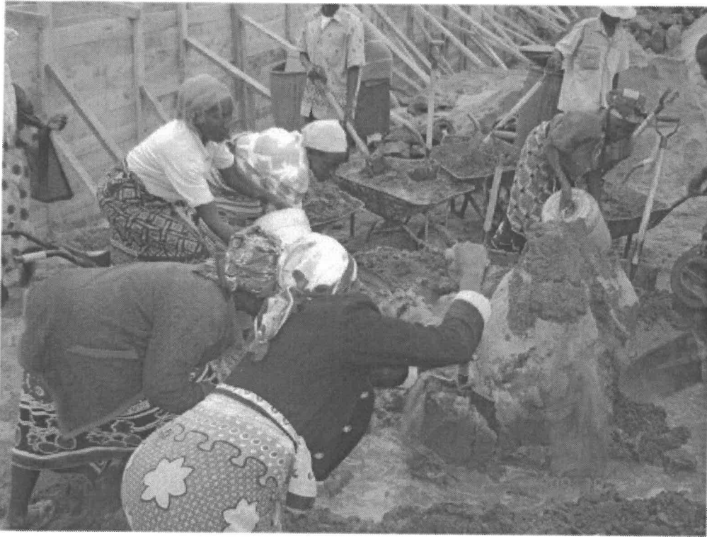
Figure 4: Community members mixing mortar at Woni Wo Tithi, Kenya
