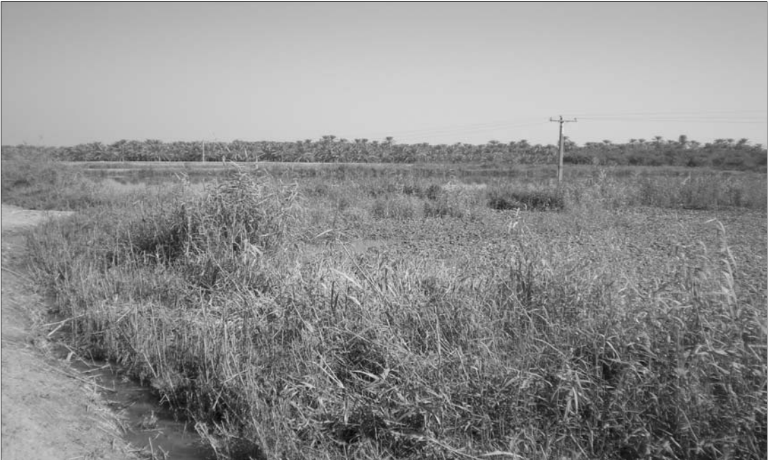
Waste stabilisation pond in Khairpur, Pakistan. The weed growth shows that even the simplest technologies will suffer if basic maintenance is neglected.
