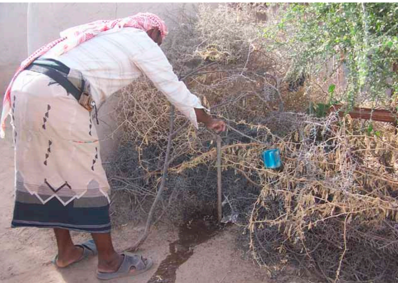
Yard connection in Yemen
