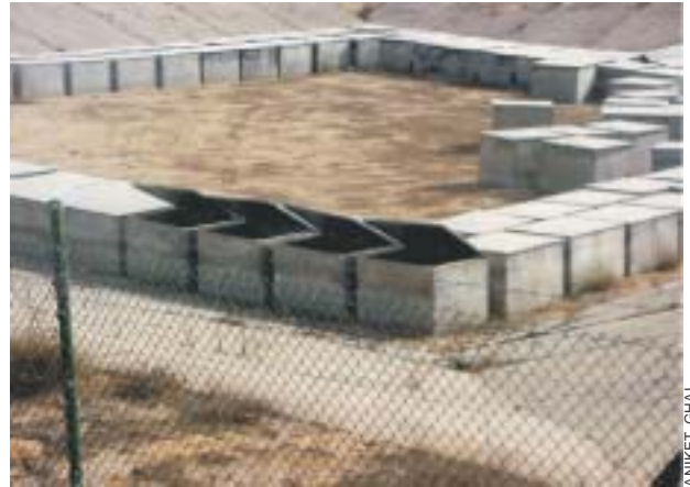
Hazardous waste temporary storage facility in Gaza
