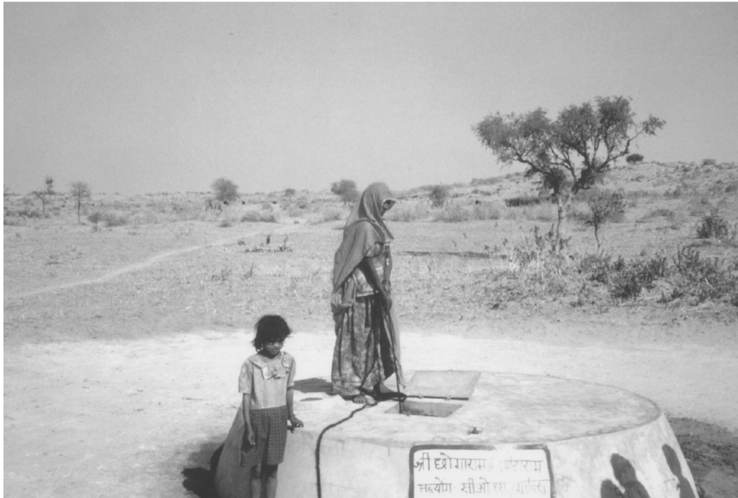
Figure 3. Photograph showing close up of taanka and extraction hatch
