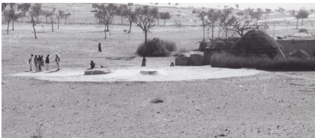
Figure 2. Photograph showing family taanka with apron for harvesting water
