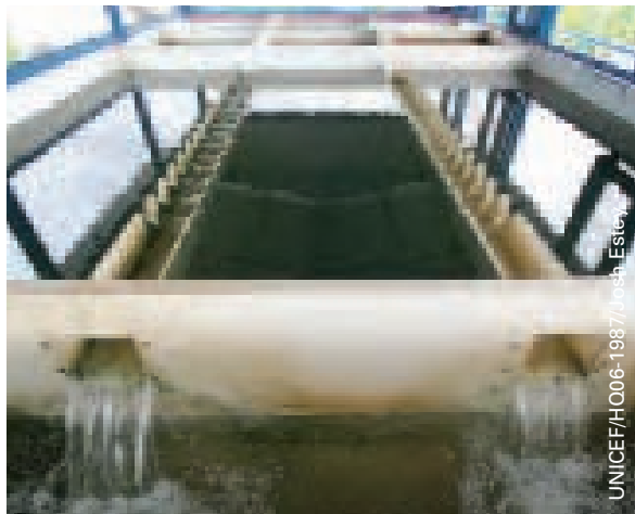
Water is processed at a UNICEF-supported water treatment plant in Siron, Aceh Province, Indonesia. The plant serves some 30,000 people still displaced by the 2004 tsunami.
