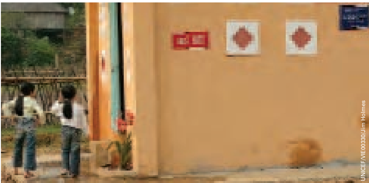
A new latrine block including child-height toilets and wash basins has been fitted at this school in a northern province of Viet Nam. UNICEF promotes latrine construction in rural and remote areas, along with promoting hand washing as a basic and easily attainable hygiene step.
