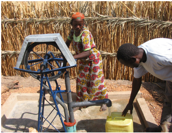
Hand drilled well equipped with locally made rope pump
