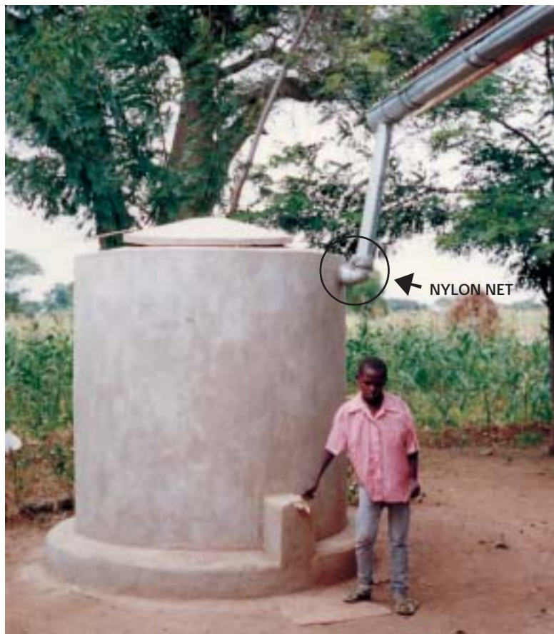
Figure 3-41: A completed 3,200-litre tank.
