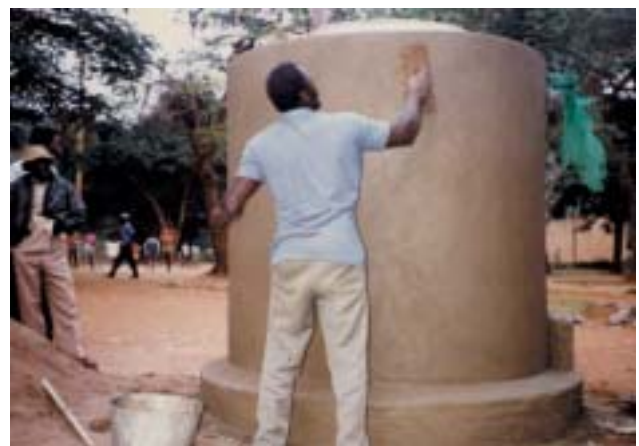
Figure 3-39: Use a sponge to smooth the tank surface.
