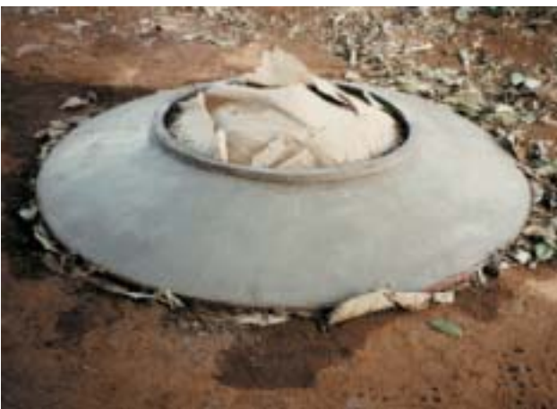
Figure 3-28: Remove the moulds after one hour. Water the cast cover for curing for at least 3 days, though again, curing for 7 days would be better.
