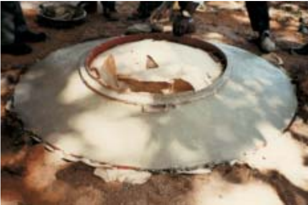
Figure 3-27: Place the 80 centimetres diameter inner mould on top of the paper-covered sand base to cast the tank mouth. Fill the space between the two moulds with the 1:2 cement mortar and fill up to the top level of the moulds.
