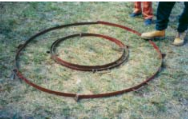
Figure 3-5: Measurements of moulds (set of 3) for the LOWER COVER of tank. Iron strips of 0.4 centimetre thick and width of 6 centimetres and 3 centimetres are used to make the moulds. Diameters of the outer and inner moulds are 162 centimetres, 87 centimetres and 80 centimetres, respectively. Detail dimensions are shown in the drawing.
