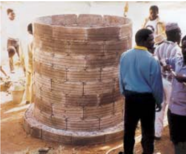
Figure 3-35: Reinforce the 8 layer-segment tank body with 0.1 centimetre diameter binding wire as shown. Insert a tap about 10 centimetres above the foundation floor. An inlet pipe is fixed onto the last layer of segment.
