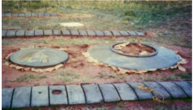
Figure 3-29: Finished segments and covers for tank.
