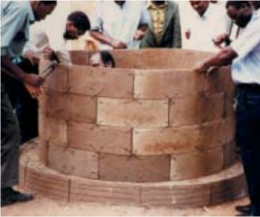
Figure 3-34: Assemble the pre-cast segments to form a tank body.
