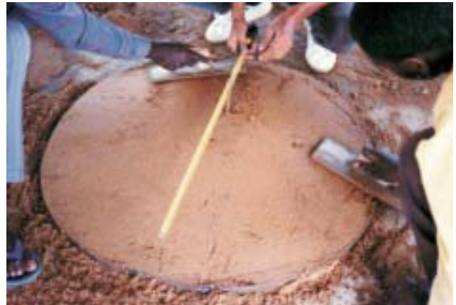
Figure 3-14: Prepare a conical sand base inside the 92 centimetres diameter inner mould with 18 centimetres height at the centre. Insert a piece of wire into the sand to mark the centre.
