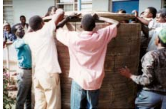
Figure 3-37: Put the cover on top of the tank after plastering the inside tank wall.
