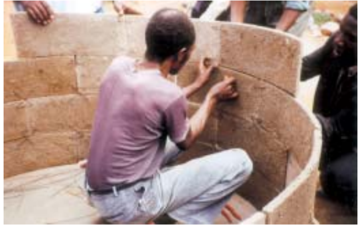
Figure 3-34: Assemble the pre-cast segments to form a tank body.
