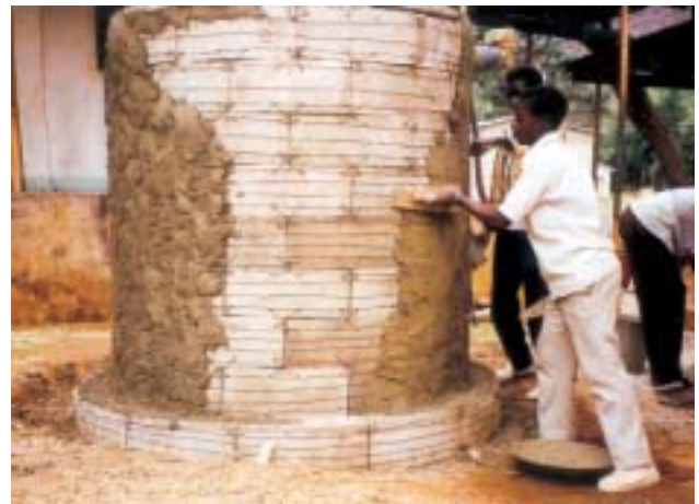
Figure 3-38: Plaster the outside wall of tank with two coatings of 1:2 cement mortar that are each 1.5 centimetres thick. Again, it is necessary to wait for a half an hour before plastering the second coating. And again, care must be taken to avoid making the mortar plastering too thick.
