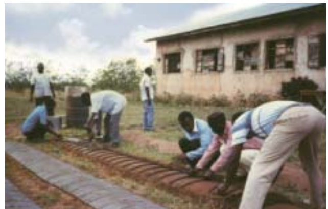
Figure 3-13: Cast cement segments for tank construction in action.
