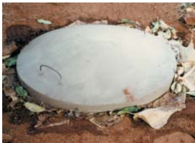
Figure 3-20: A finished upper cover with handles.
