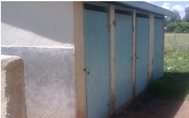
Photo 2: Angra boys latrine and urinal
