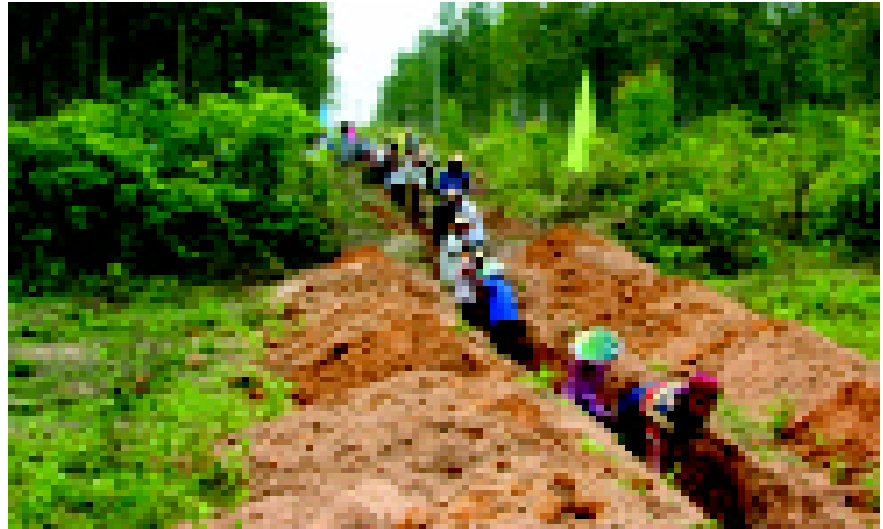
Community labor contribution: digging of trench for laying pipeline
