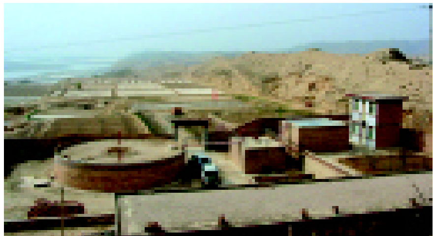
Large water supply plant in Gansu province
