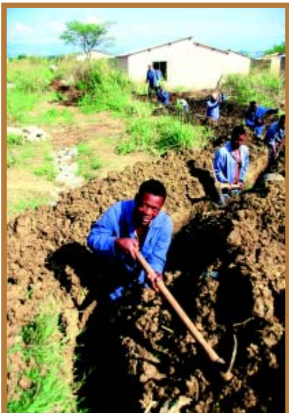
Community members dig trenches to lay water pipes, South Africa.
